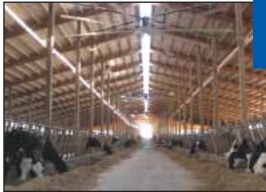
Gold Top Farms in Maine (left) is saving 90,000 kilowatt hours of electricity annually with high-volume, low-speed fans in its barn. Above, an anaerobic digester converts cow manure into methane gas, which in turn produces electricity.
