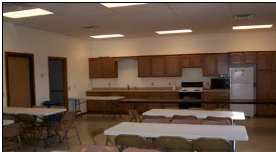
Community Room Cabinets
