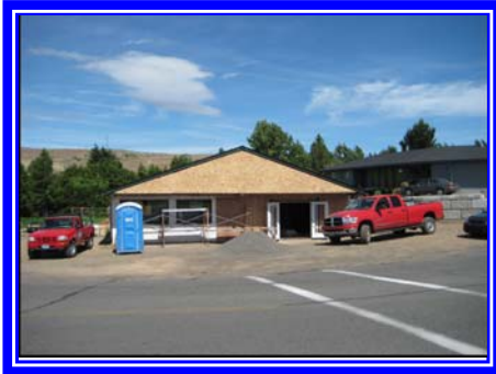
Remodeling of Building
