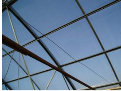
NEW ROOF MATERIAL
