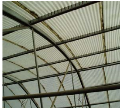
ROOF OF OLD FIBERGLASS GREENHOUSE
