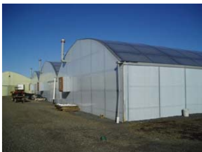
NEW DOUBLE WALL LEXAN ON ROOF & SIDES
