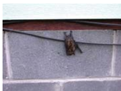
Bat found roosting on outside of structure
