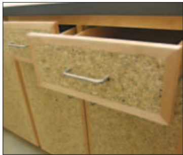
TOP DRAWERS: Drawers and cabinets inside the CTS building are made of compressed sunflower seed agri-board.
