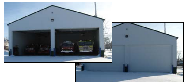
Pictured above is the Dana Fire Protection District (FPD) facility in La Salle County. Dana FPD received a $105,000 loan and $24,194 grant to expand and build an addition to their fire house.
