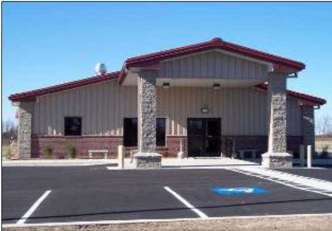
USDA Rural Development Community Facilities Grant funds provided unincorporated Franklin, KS with this community center after a tornado destroyed the previous facility.
