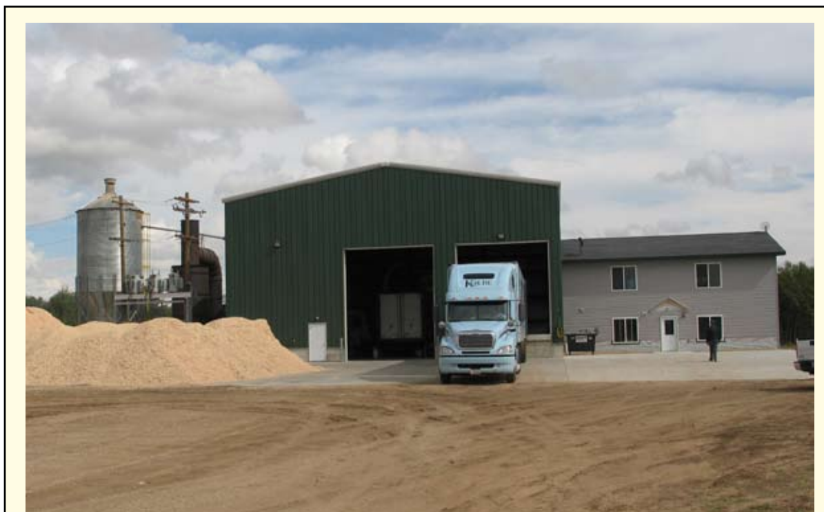
Isabella Pellet's manufacturing facility is an example of taking an abundant local resource - in this case, lumber waste - and utilizing it to promote energy independence and create jobs.
