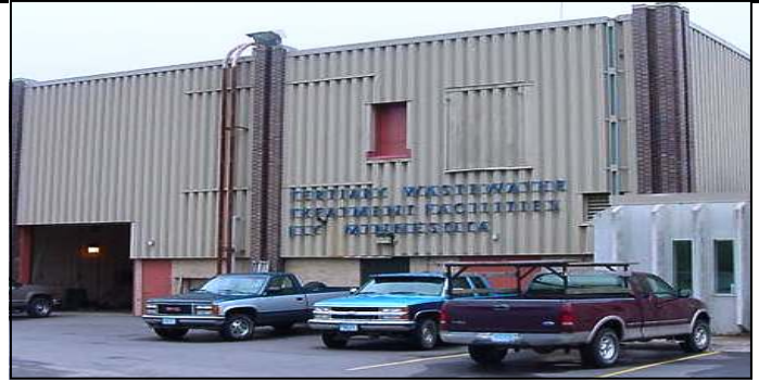
The outside of the wastewater treatment building in Ely.
