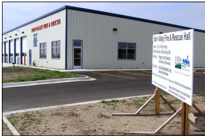
This new fire hall in Eden Valley was built using USDA Rural Development’s Rural Economic Development Loan and Grant program and its Community Facilities Program.
