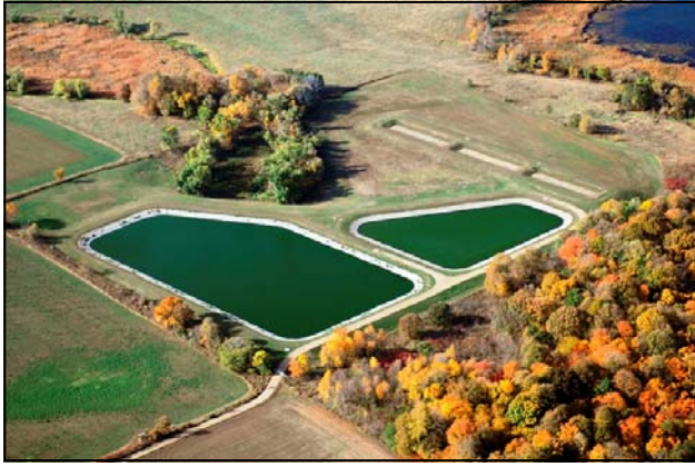
Here is an overhead view of the new wastewater ponds constructed in Dent using Rural Development financing.
