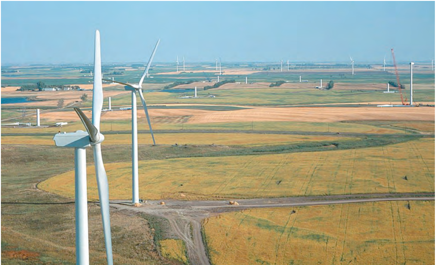
Basin Electric Cooperative already generates 136 megawatts (MW) of electricity at wind farms such as this, and will be expanding with an additional 300 MW (see related article, page 31). Photos courtesy Basin Electric Cooperative
