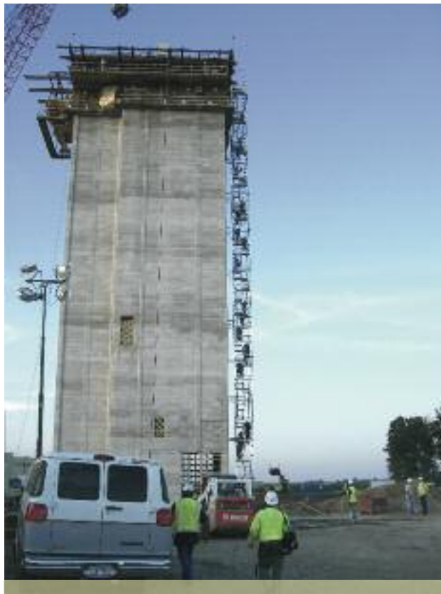
New Vision Co-op’s feed mill in Magnolia, Minn., during construction. The grain elevator at the $12.6 million facility is expected to open by November, with the feed mill to be in operation by June.
