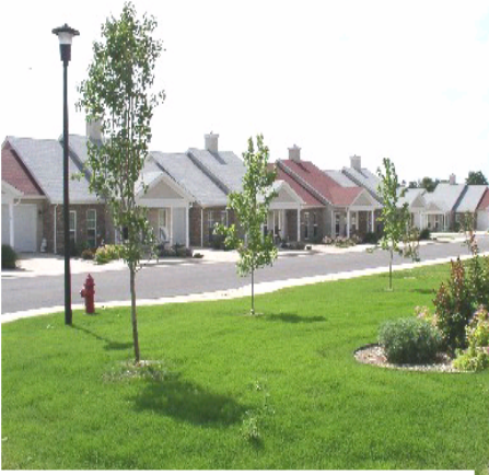
Picture 1, Park West Apartments These beautiful, 36 multi-family rental units in sought-after Mountain Home, Arkansas, were built for persons 55 and older. The average rent of $490 per month, including utilities, is an affordable option for senior living in this rural community.
